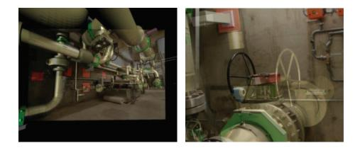
**Figure 1.12** AR can be used for discrepancy analysis in industrial facilities. These images show still frames overlaid with CAD information. Note how the valve on the right-hand side was mounted on the left side rather than on the right side as in the model. Courtesy of Nassir Navab.
